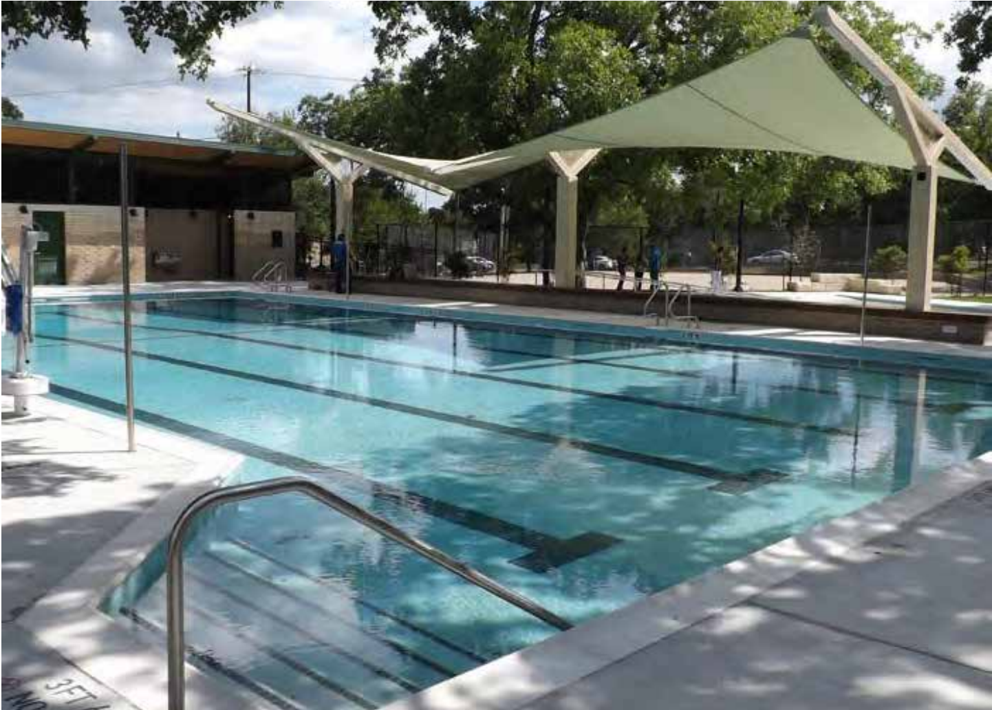
West Enfield Pool Renovation | Wimberley, TX
